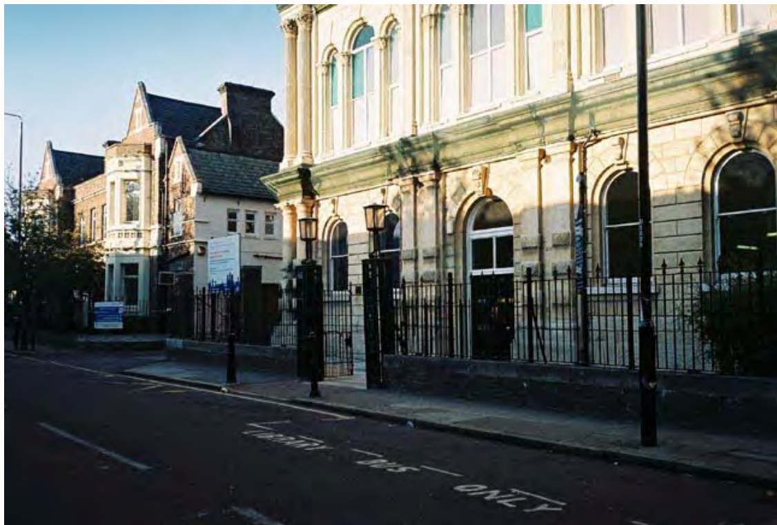
Figure 3: A current view of Bancroft Road Buildings, E1, showing from the left, the former Marriage Registry Office; the entrance to Mile End Hospital, and the Public Archives and Local Studies Library, standing in front of Queen Mary and Westfield College.
